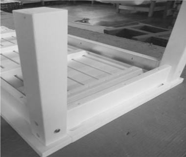
Place Table Top face down on a flat clean surface. Place Leg Assembly upside down on each side of Table Top aligning pre-drilled holes and facing the Aluminum Cleat inside the Table Top (Left Picture). Attach using (2) 3" Hex 1/4" Lags. Repeat process on other side. (Right Picture)
