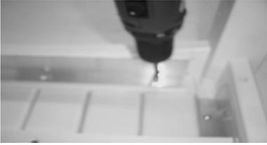
Attach Short Apron Aluminum, which is pre-assembled on Leg Assembly to Table Top using (3) 3/4" Pan Head Screws. (Left Picture) Repeat process on other side.
